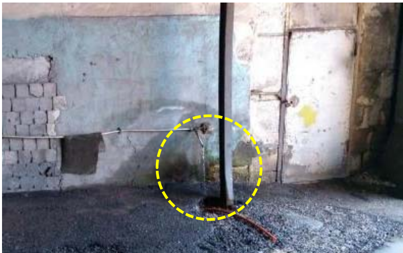
Figure 4-9. Inefficient water use at the bus washing station of Nor Nork depot
