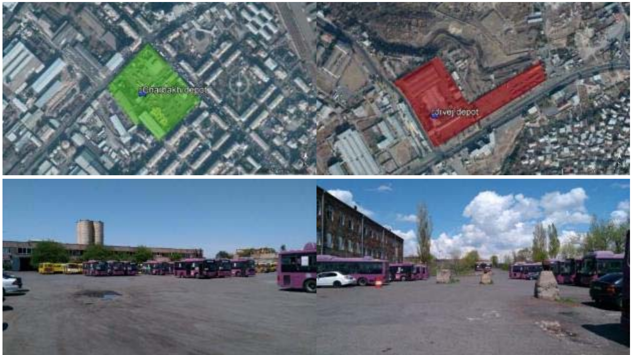
Layout and general view of Charbakh bus depot
