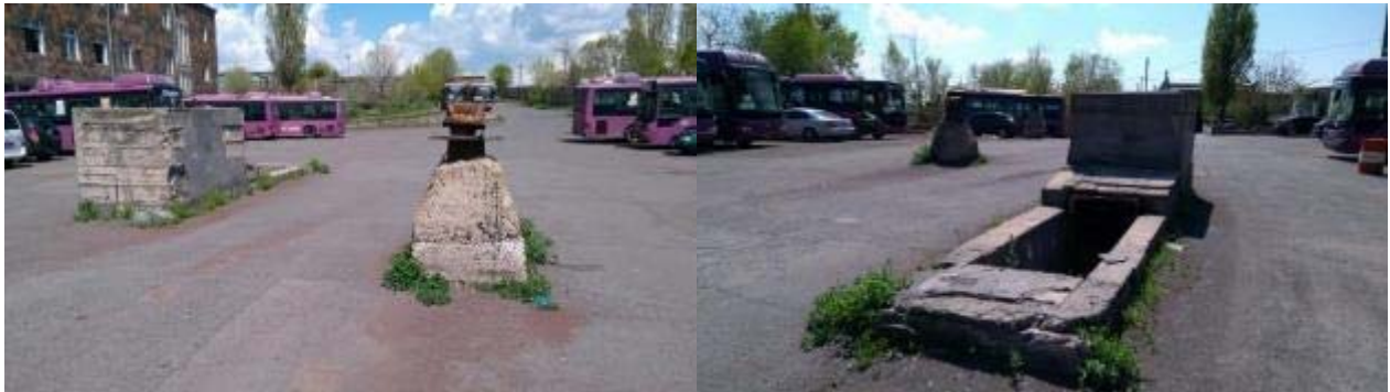
Figure 4-19. Emergency shelter in Nor Nork (Jrvej) depot
